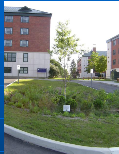
Figure 11-P4-1 Earthen Surface Sand Filter
